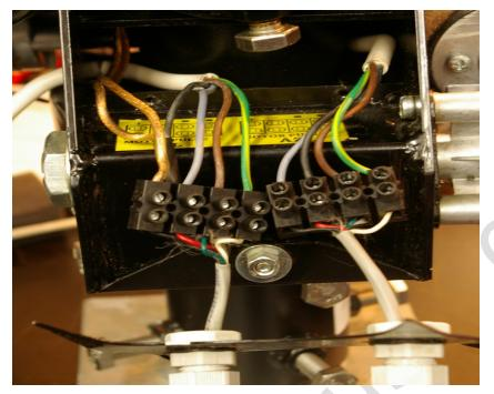
On the RAS and BIG-RAS Rotator, remove cover from the rotator and pull out the two 4 pin terminal strips. The Elevation terminal strip is on the left of the above picture and the Azimuth is on the right. Each terminal strip has pin 1 on the left and pin 4 on the right.
